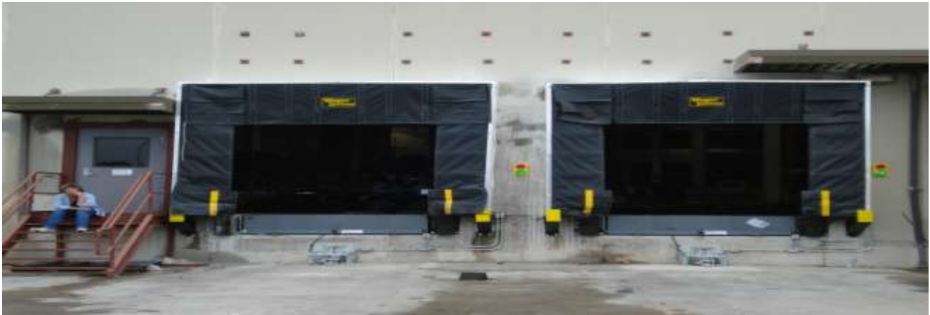
Installation of (2) dock Doors 9 x 10 – Steel work – Steel stairs
